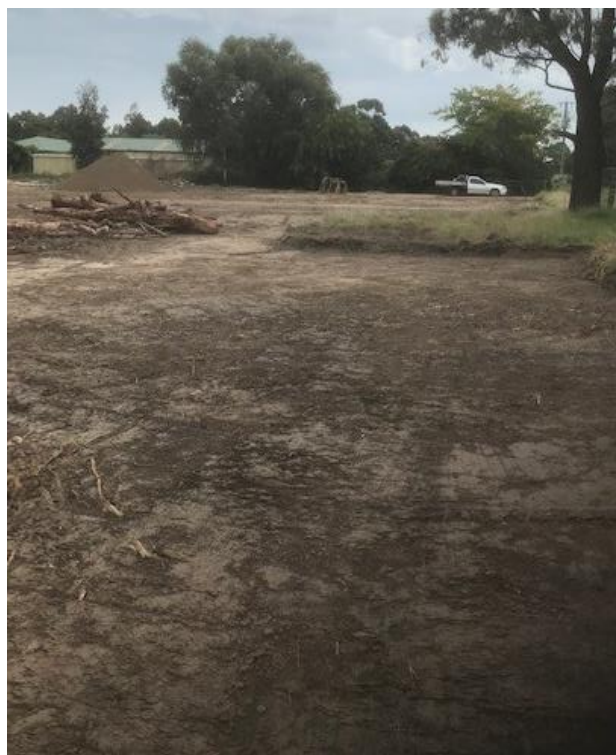
Figure 3: Level 1 Stripping Inspection - 22/03/2024
