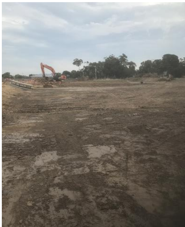
Figure 2: Level 1 Stripping Inspection - 22/03/2024
