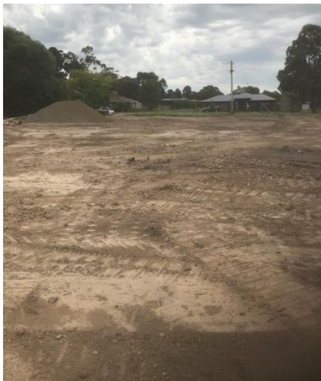
Figure 1: Level 1 Stripping Inspection - 22/03/2024
